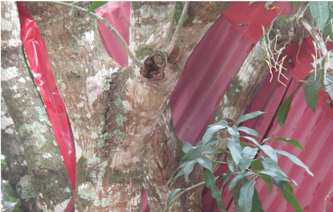
The damage roof of one of the buildings at the school.
