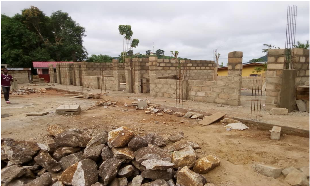
The new building under construction.
