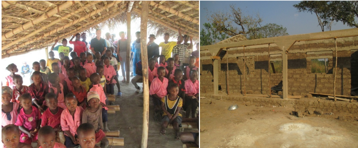
At shekuya , it was pathetic and shocking for the North American to see this place been used as a classroom. But on the right is the new structure World renew through CES is building to provide a good reading and learning environment for the pupils in Shekuya village.
